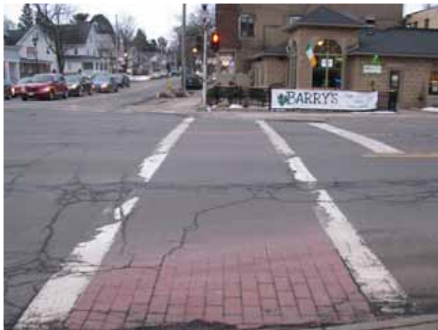
▲ Crosswalk at four-corners
