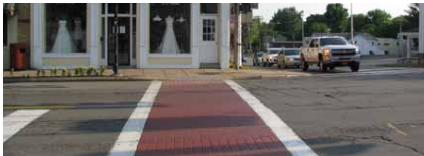
Textured crosswalk at four-corners ▼
